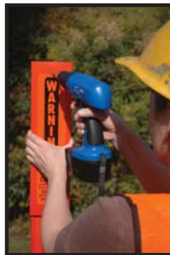
Enhancer is supplied with holes that can be used as a template to field drill existing marker.
